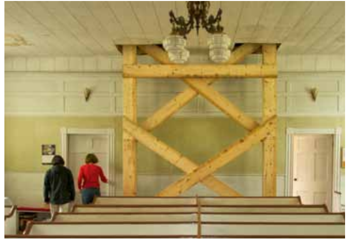
Inside the Troy Union Church undergoing renovations.
